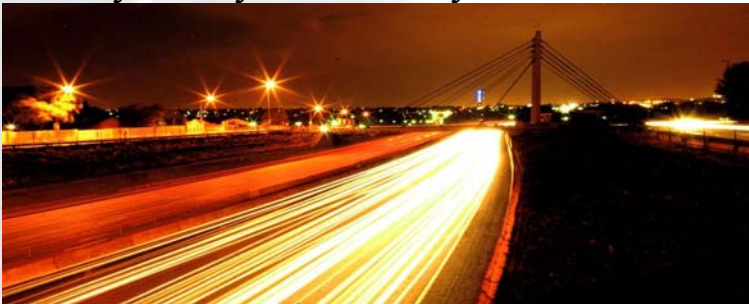
Nelson Mandela bridge silhouette
