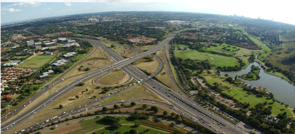
City Road infrastructure
